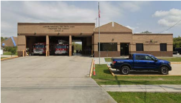
Image #1: Station 40 located at 2385 Jean Lafitte Boulevard in Lafitte
