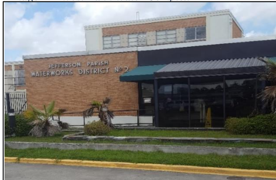
Image 11- West Bank Water Complex
